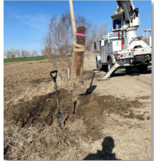
*Drill rig crane lowering monument into position after digging hole.*
