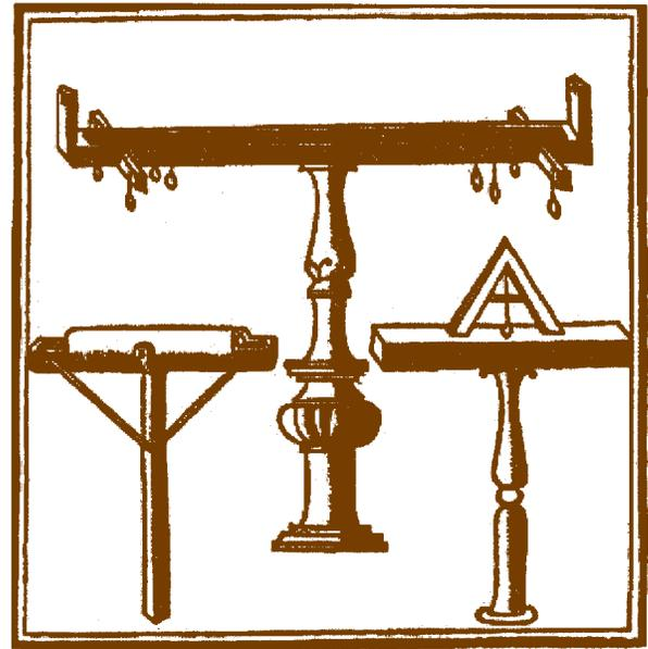
Figure 7. Alternate, older version of Chorobates. A scaled down demonstration model Fra Giovanni Jocundus, AD 1511
