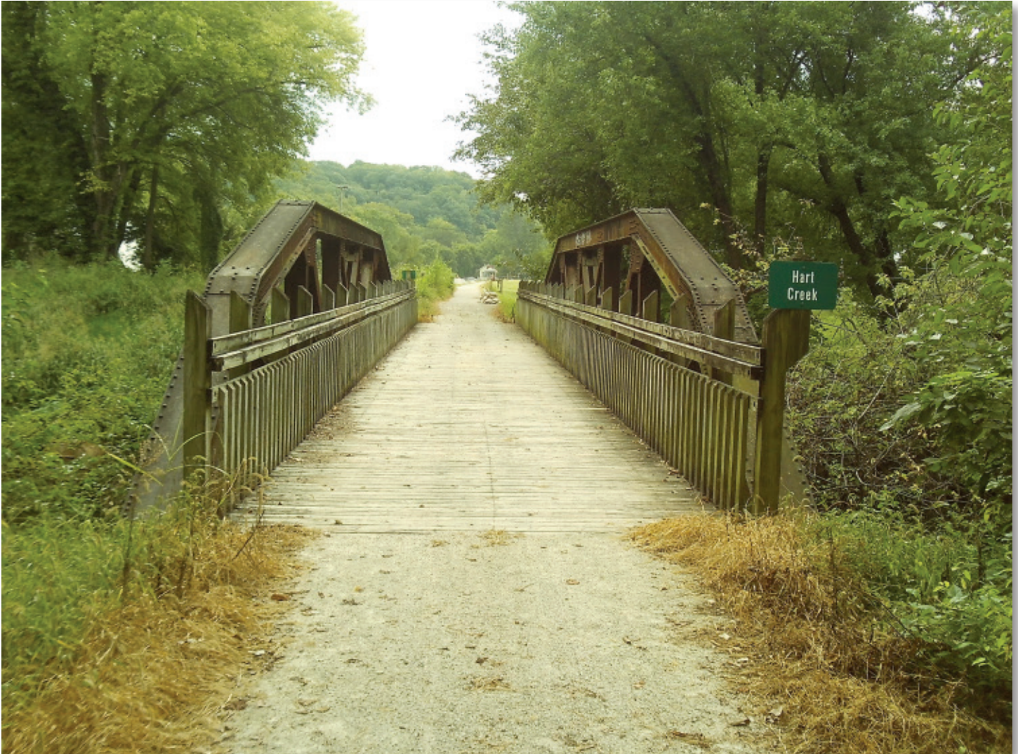
The Katy Trail Hart Creek Bridge in southern Boone County at Hartsburg.
